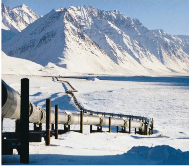
Figure 3.1: Trans Alaskan Pipeline system (TAPS) extended over 800 miles.
