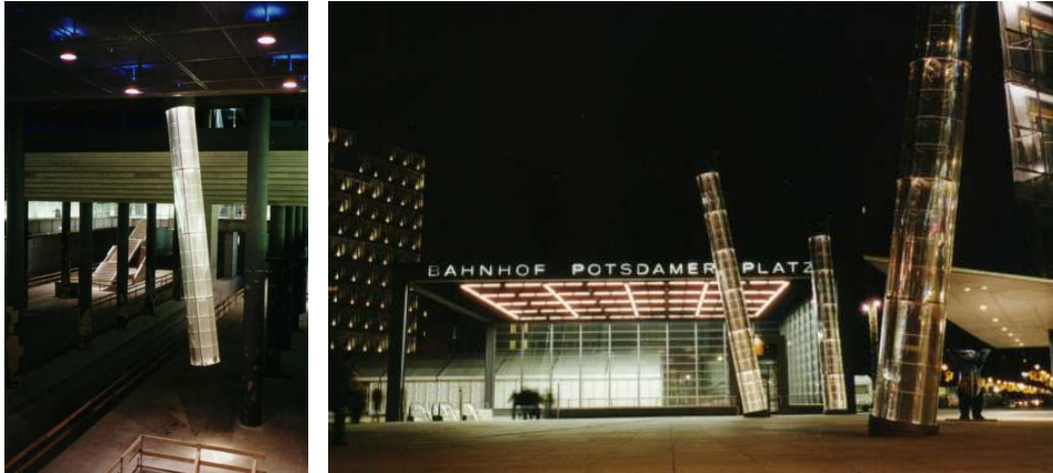
Figure 4.22: Lightpipes in vertical configuration at Potsdamer Platz subway station, Berlin. The pipes conduct daylight to the subway platforms below (left). At night they conduct artificial light from lamps mounted within (right).
