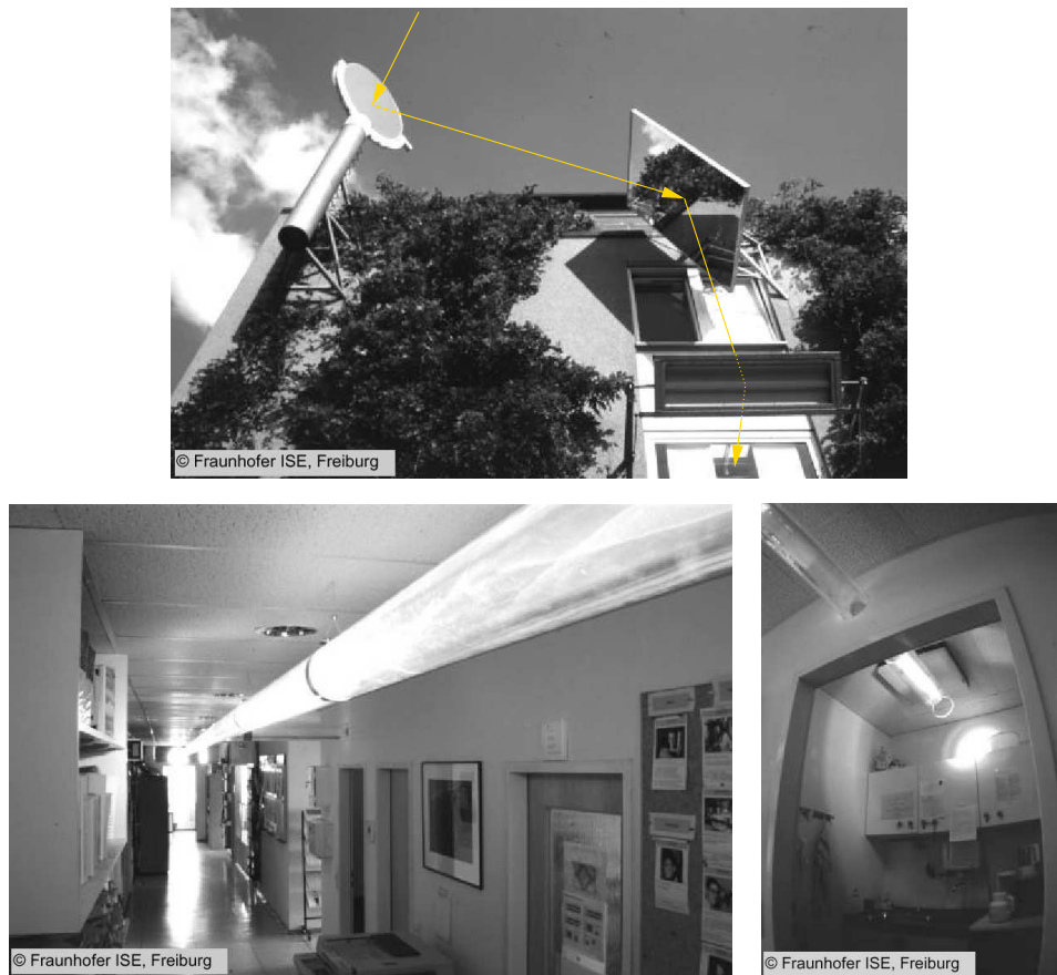
Figure 4.21: Lightpipe installation in 1st floor corridor at Fraunhofer ISE. Sunlight is directed into the pipe via a heliostat and two fixed mirrors (top). Daylight is then conducted by the pipe's prismatic foil through the corridor (left) and directed into rooms lacking windows (right). Images reproduced from [EGW98].
