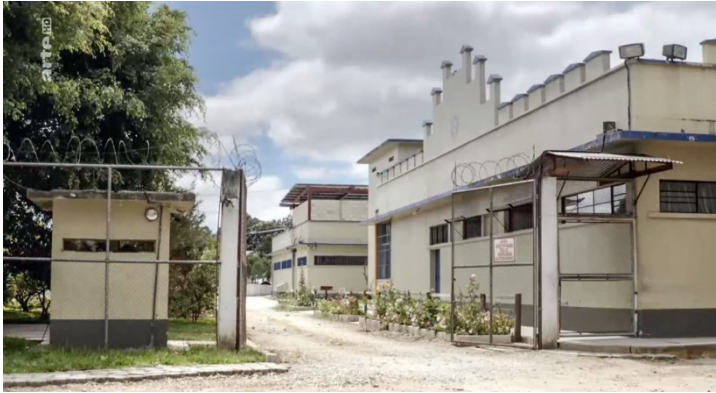
Fig. 4: The transformation of the exterior of the AHPN ( Guatemala, les disparus : 0:39:31) 75
