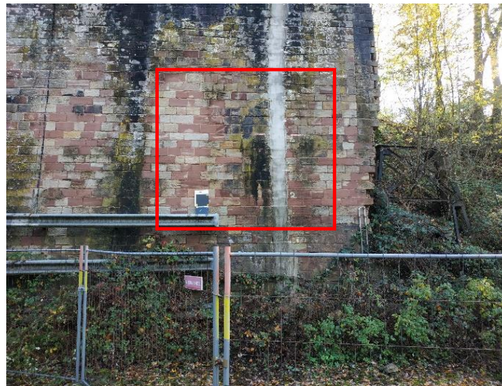
Figure 5. Overview of the wall structure under test. The rectangle shows the approximate view of the LWIR camera.
